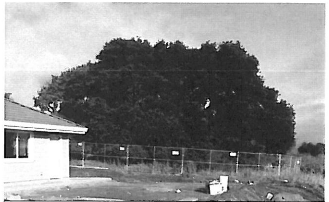
Chain link fence is preferable to orange plastic fencing to protect oaks during construction. Photo courtesy: HortScience, Inc.
