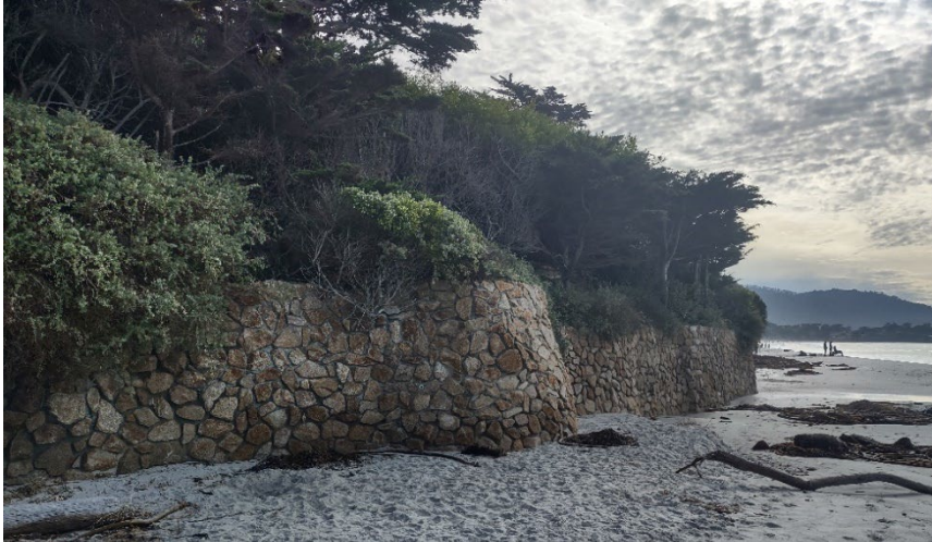
Figure 26. Privately owned seawall near Pescadero Canyon.
