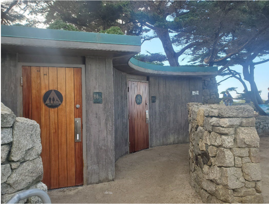
Figure 19. Restroom at Santa Lucia Avenue.
