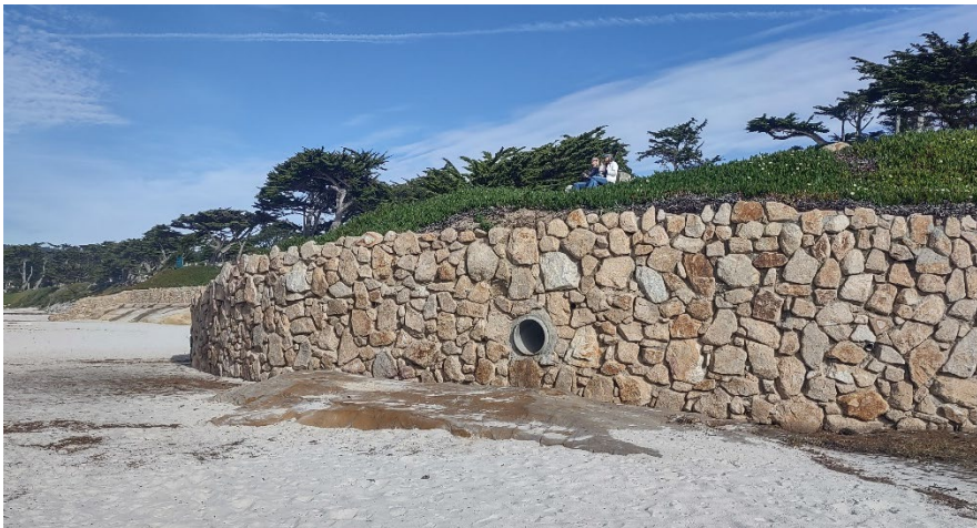
Figure 20. Stormwater drainage near 13th Avenue.
