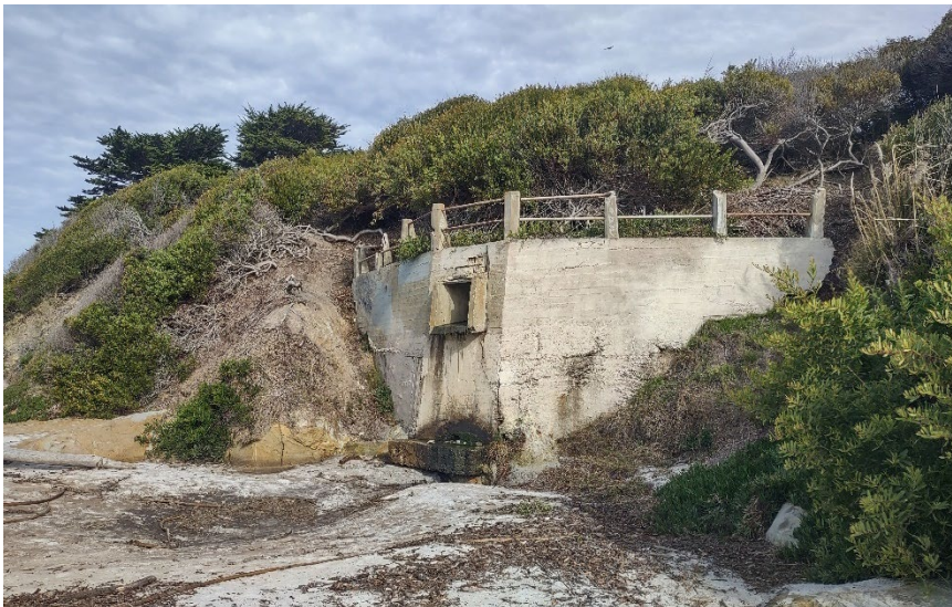
Figure 25. Seawall and outfall just south of the 4th Avenue Stairway.
