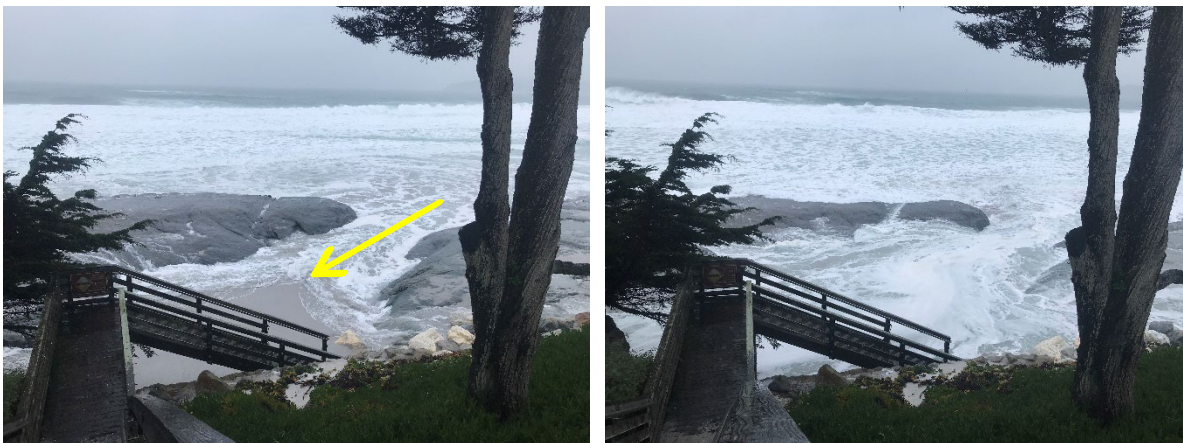
Figure 6. Focusing of water flow between the gap in the sandstone formation. This leads to a piling up of water in the gap and subsequently higher erosion. Location: Stairs at northern end of 10th Avenue. Source: City of Carmel, January 2023
