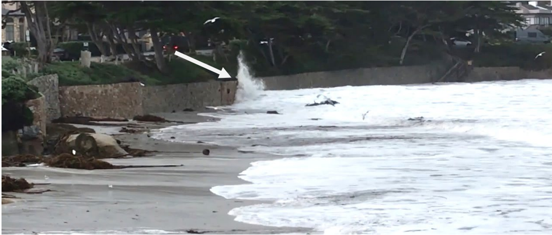
Figure 3. Wave overtopping on a Carmel seawall (see arrow). Note the directional wave and splash along the wall. Source: City of Carmel January 5, 2023
