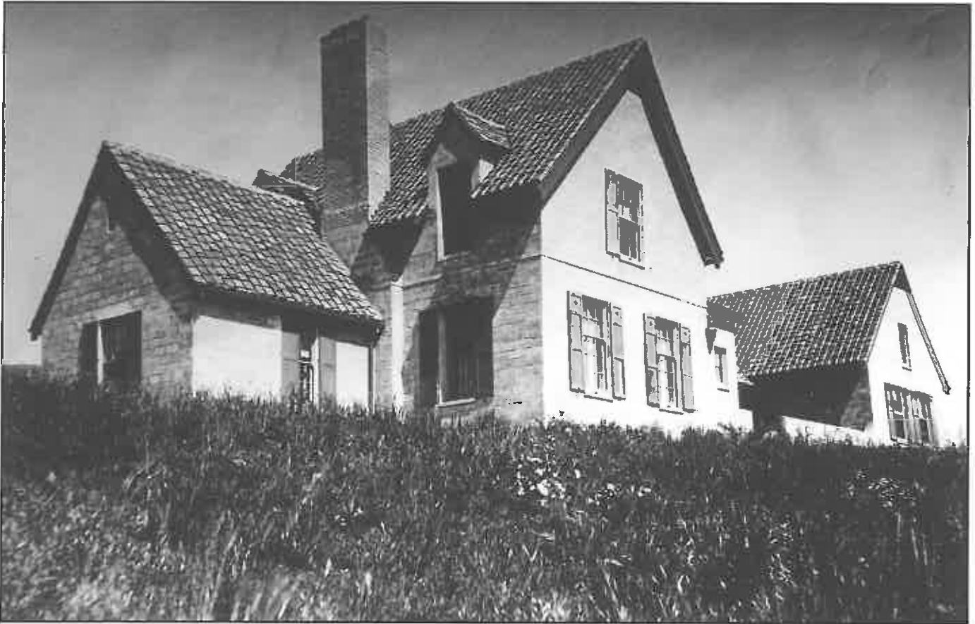
Figure C-8. South elevation looking northeast by Carmel photographer Lewis Josselyn, circa 1926 ( Courtesy: Estate of Fred Ruhl ).
