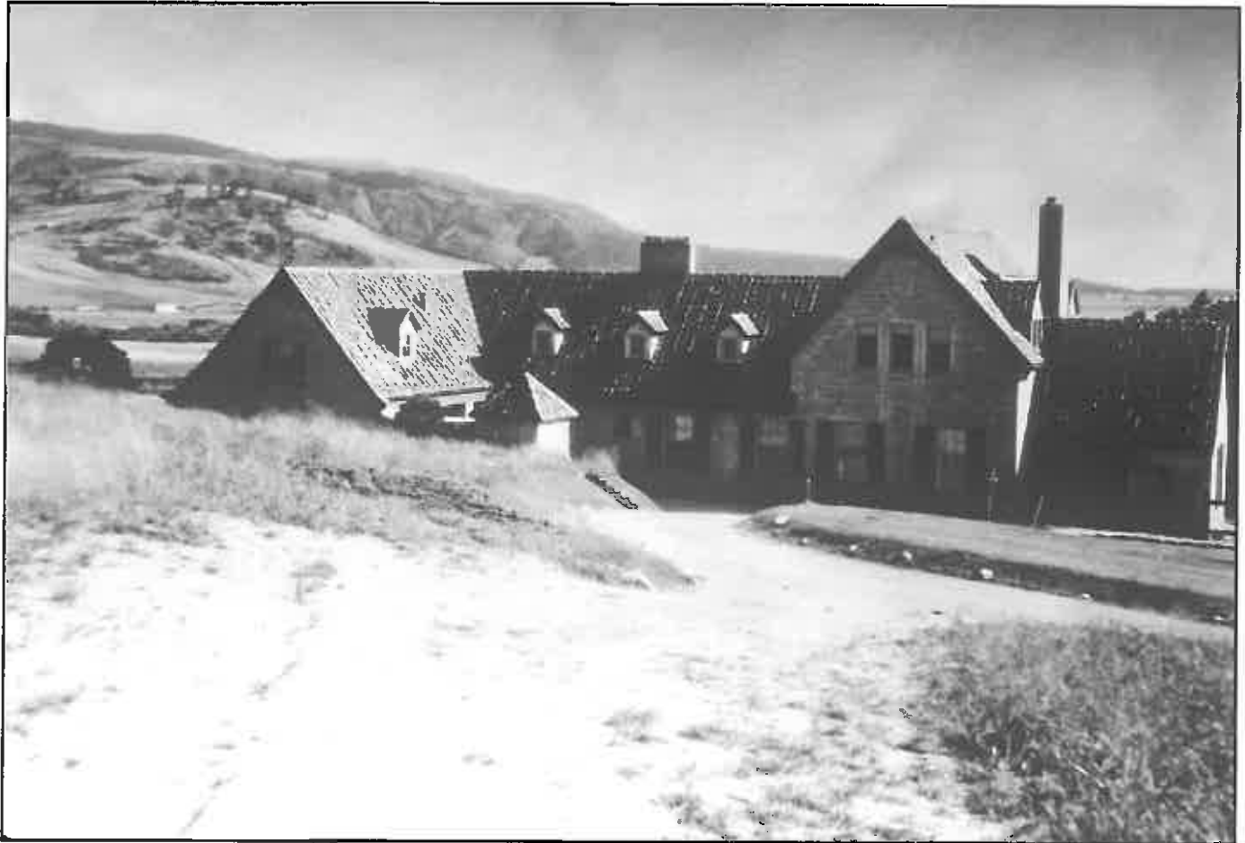
Figure C-3. North elevation looking southeast by Carmel photographer Lewis Josselyn, circa 1926 ( Courtesy: Estate of Fred Ruhl ).
