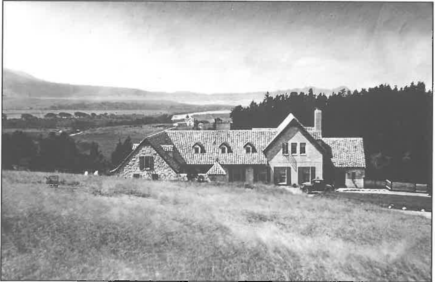
Figure C-1. North elevation looking south by Carmel photographer Lewis Josselyn, circa 1926 ( Courtesy: Estate of Fred Ruhl ).
