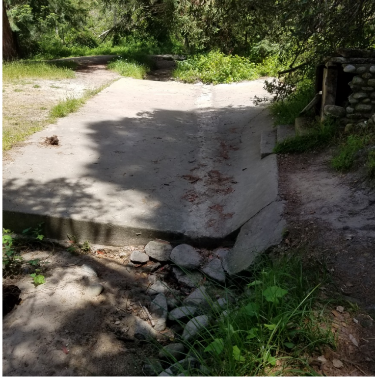
Photo #2: Looking upstream at Site #4, Concrete Ford.
