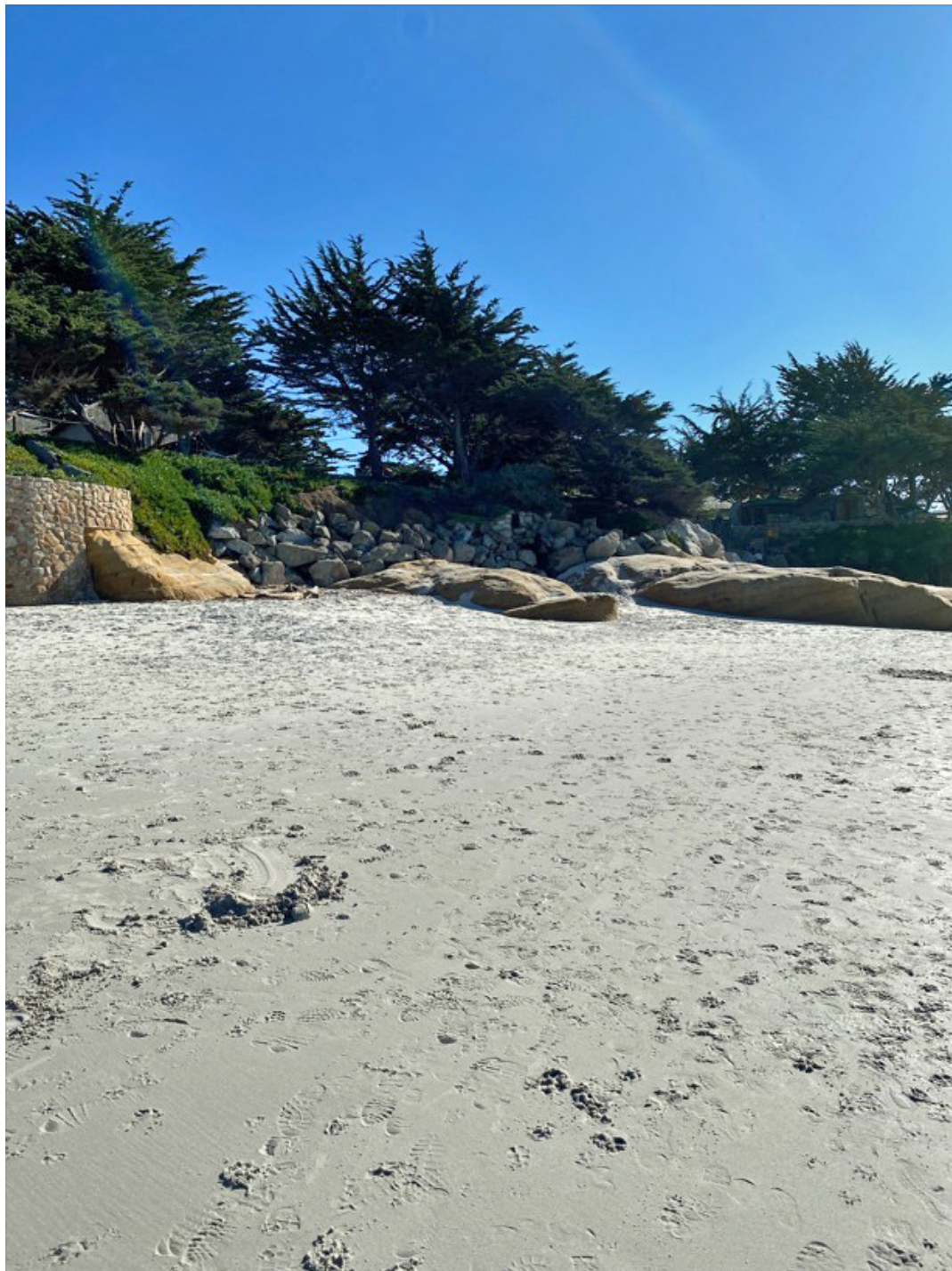
Photograph 16: Showing Revetment R1 on January 30, 2023
