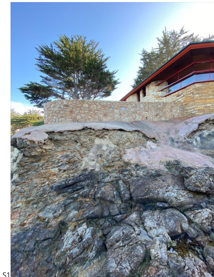
Photograph 1: Privately Owned Seawall S1 on December 22, 2022
