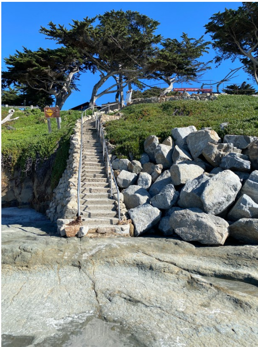
Photograph 57: Showing Stairway ST5 on January 30, 2023
