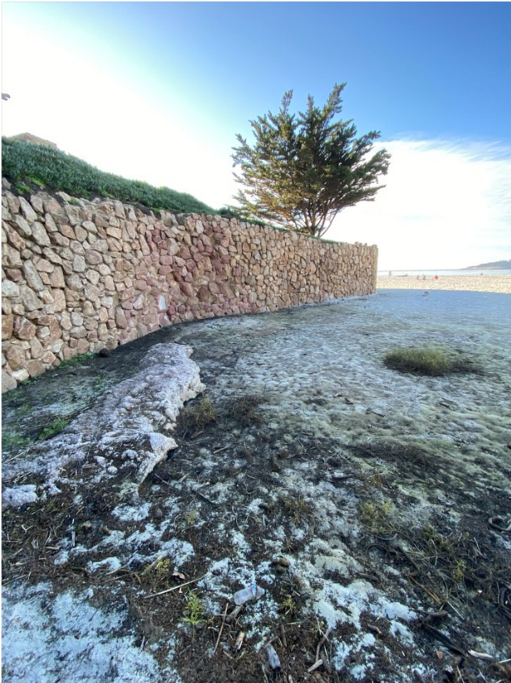
Photograph 22: Southern End of Seawall S3 on December 22, 2022
