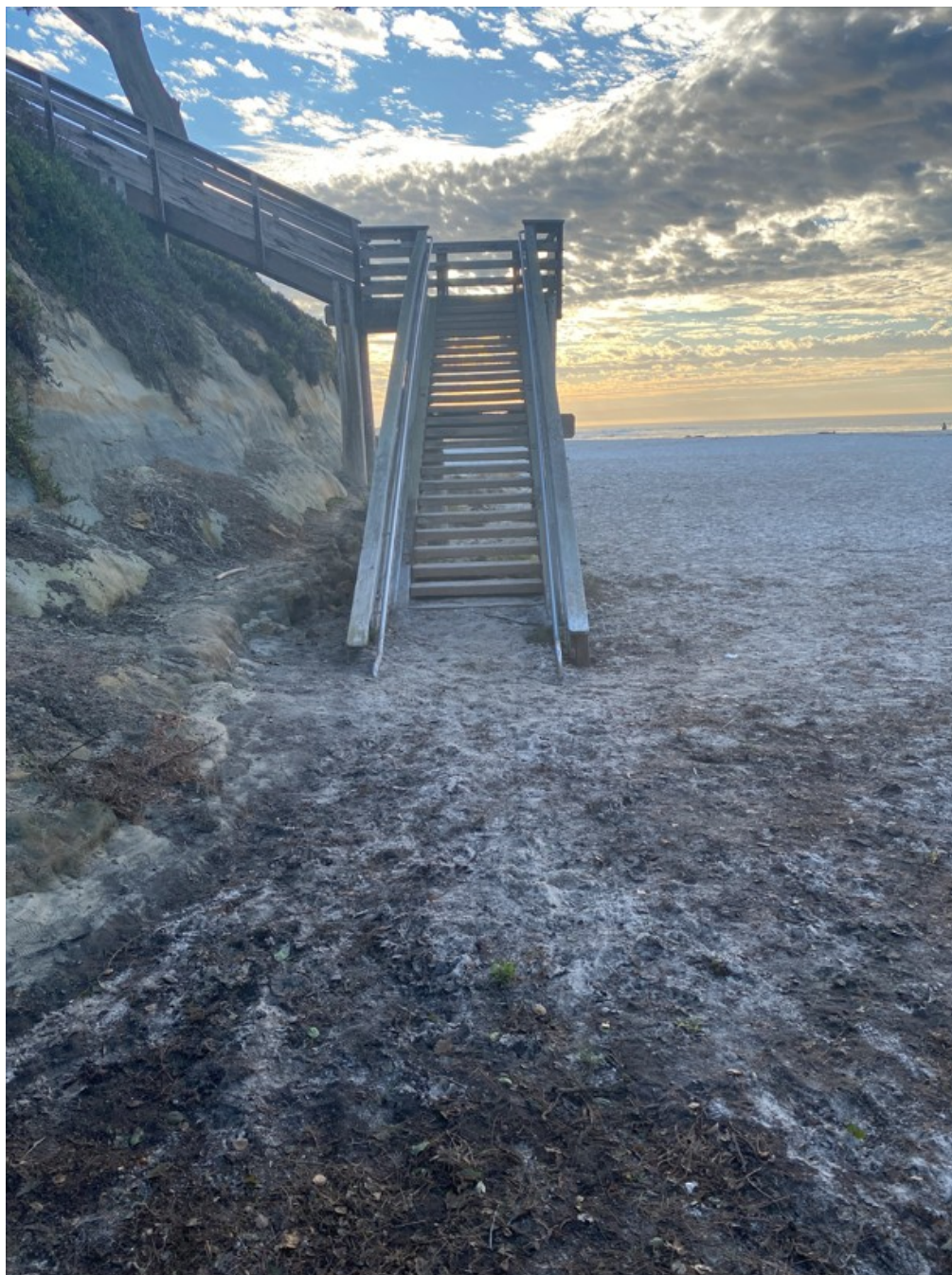
Photograph 40: Showing Base of Stairway ST4 naturally buried in beach sand on December 22, 2022
