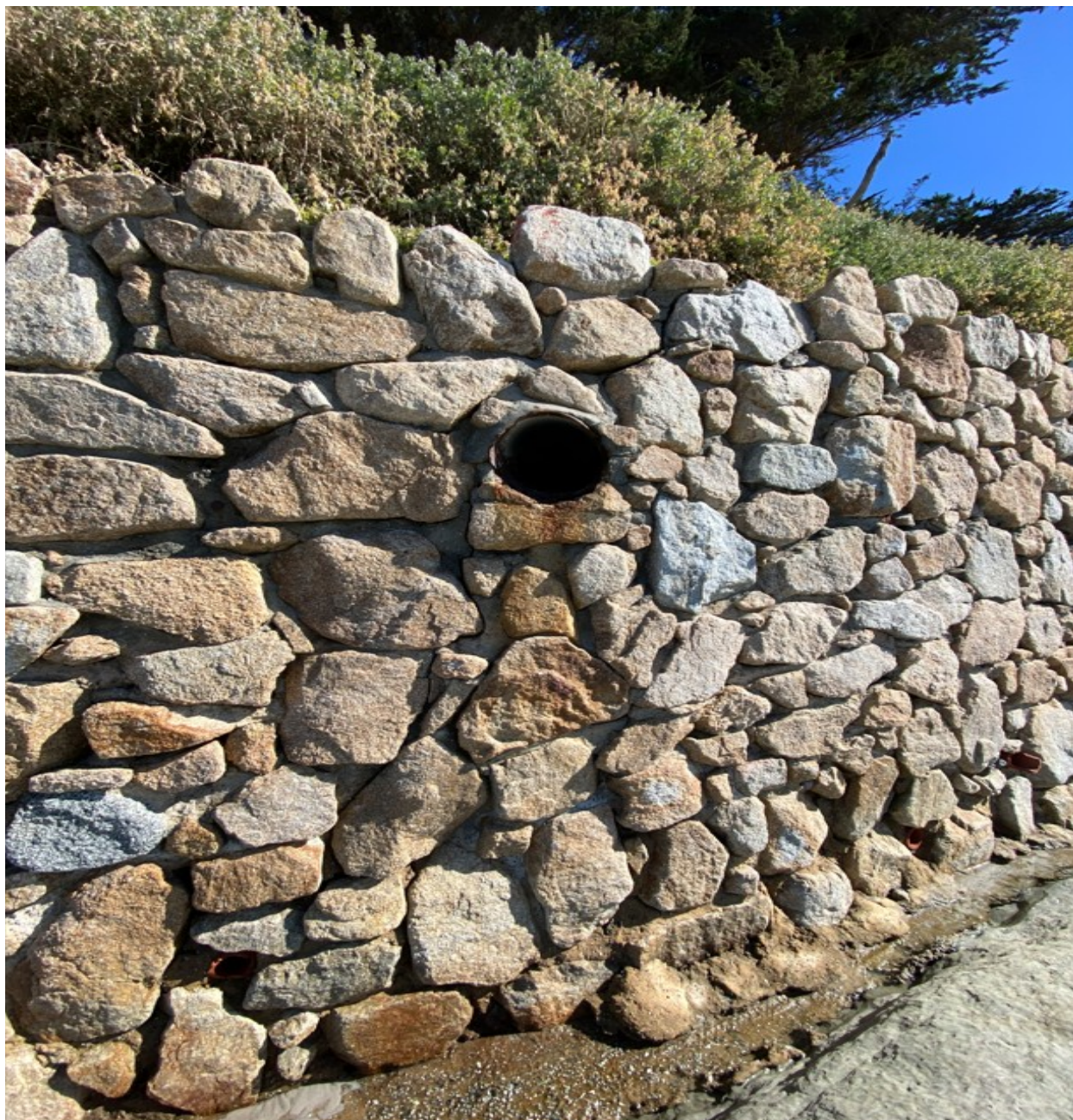
Photograph 72: Storm Drain in Seawall S7 on January 30, 2023
