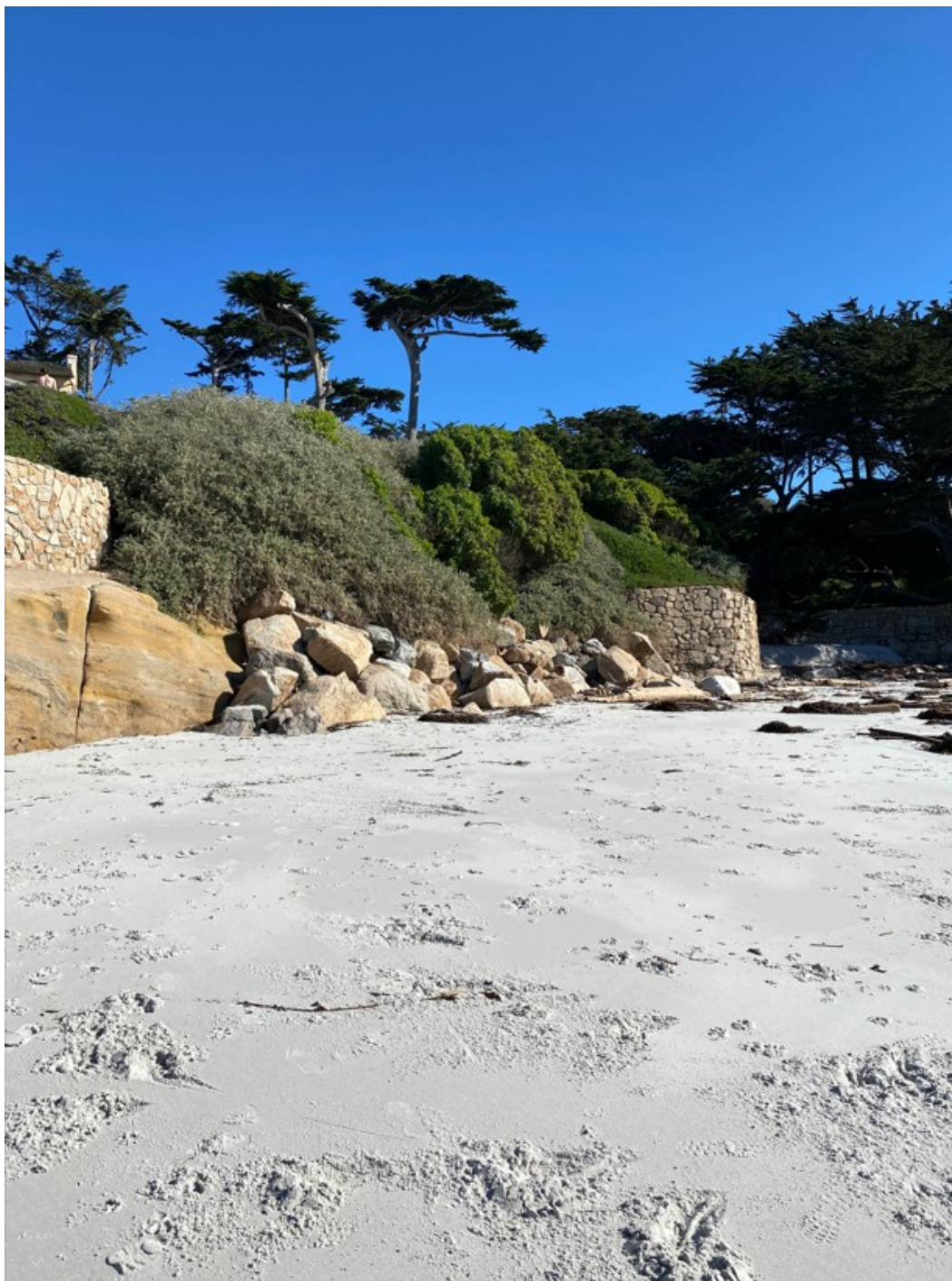
Photograph 32: Showing Revetment R2 between Seawalls S3 and S4 on January 30, 2023
