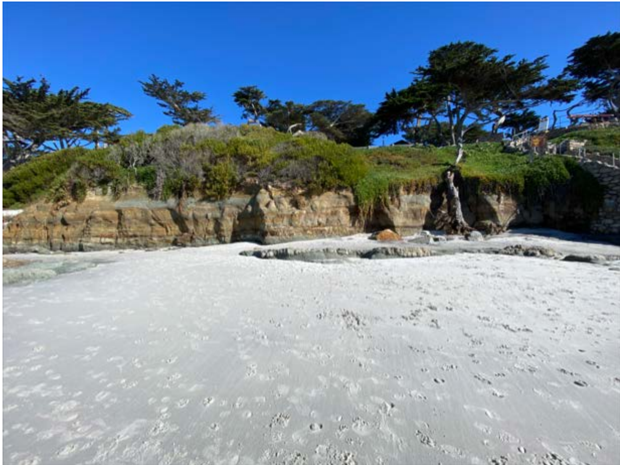
Photograph 59: Showing Bluff South of Retention R4 on January 30, 2023
