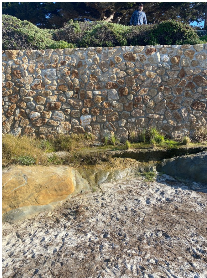
Photograph 11: North End of Seawall S2 on December 22, 2022
