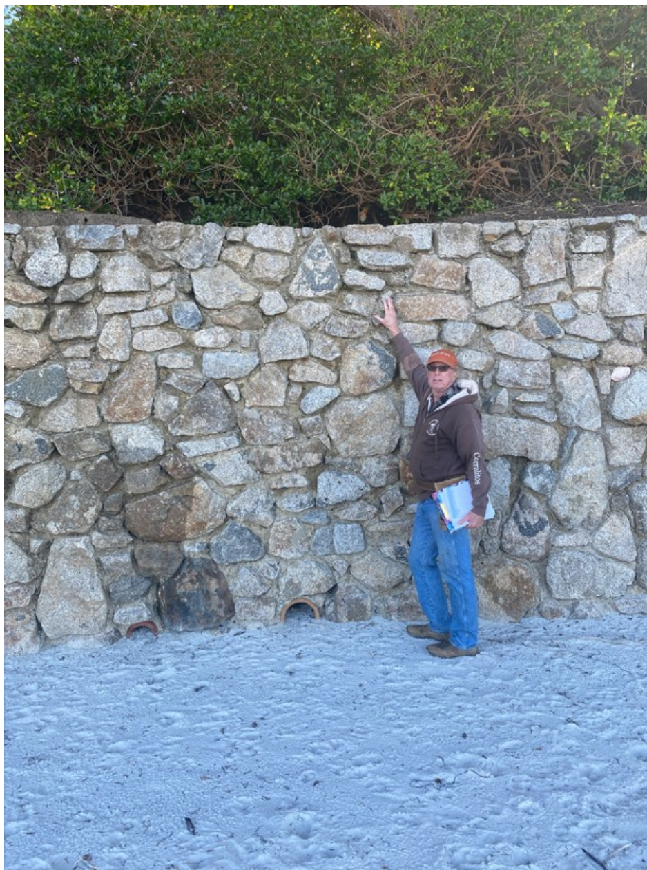
Photograph 9: Seawall S2 on December 22, 2022
