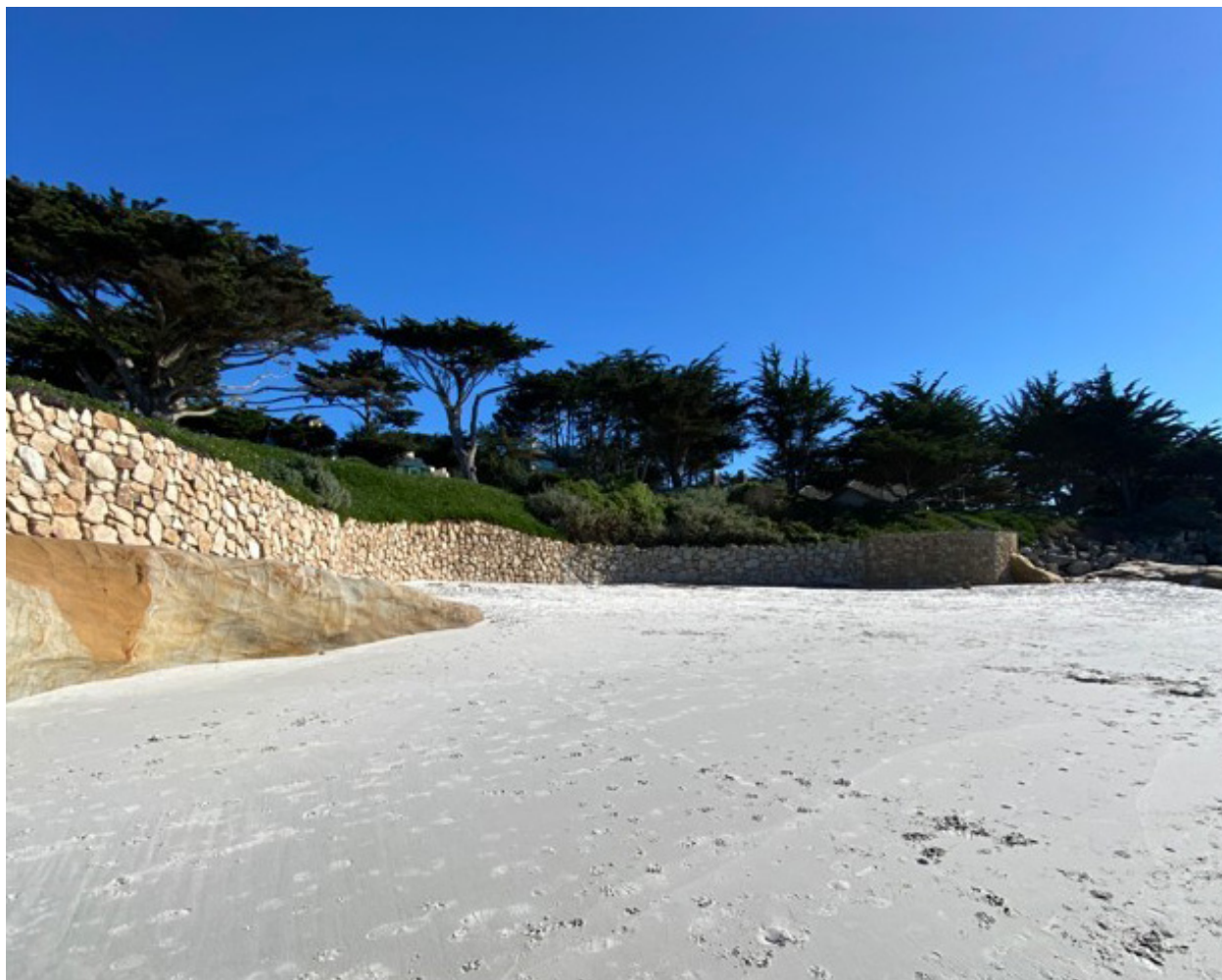
Photograph 35: Showing Seawall S4 on January 30, 2023
