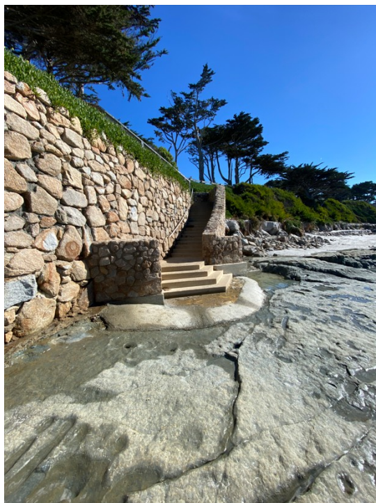
Photograph 66: Stairway ST6 Well Founded in Bedrock on January 30, 2023
