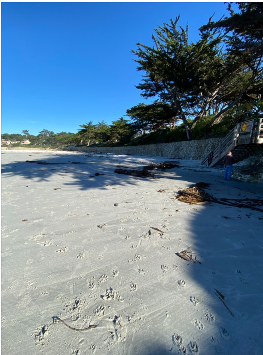
Photograph 3: Seawall S2 on December 22, 2022
