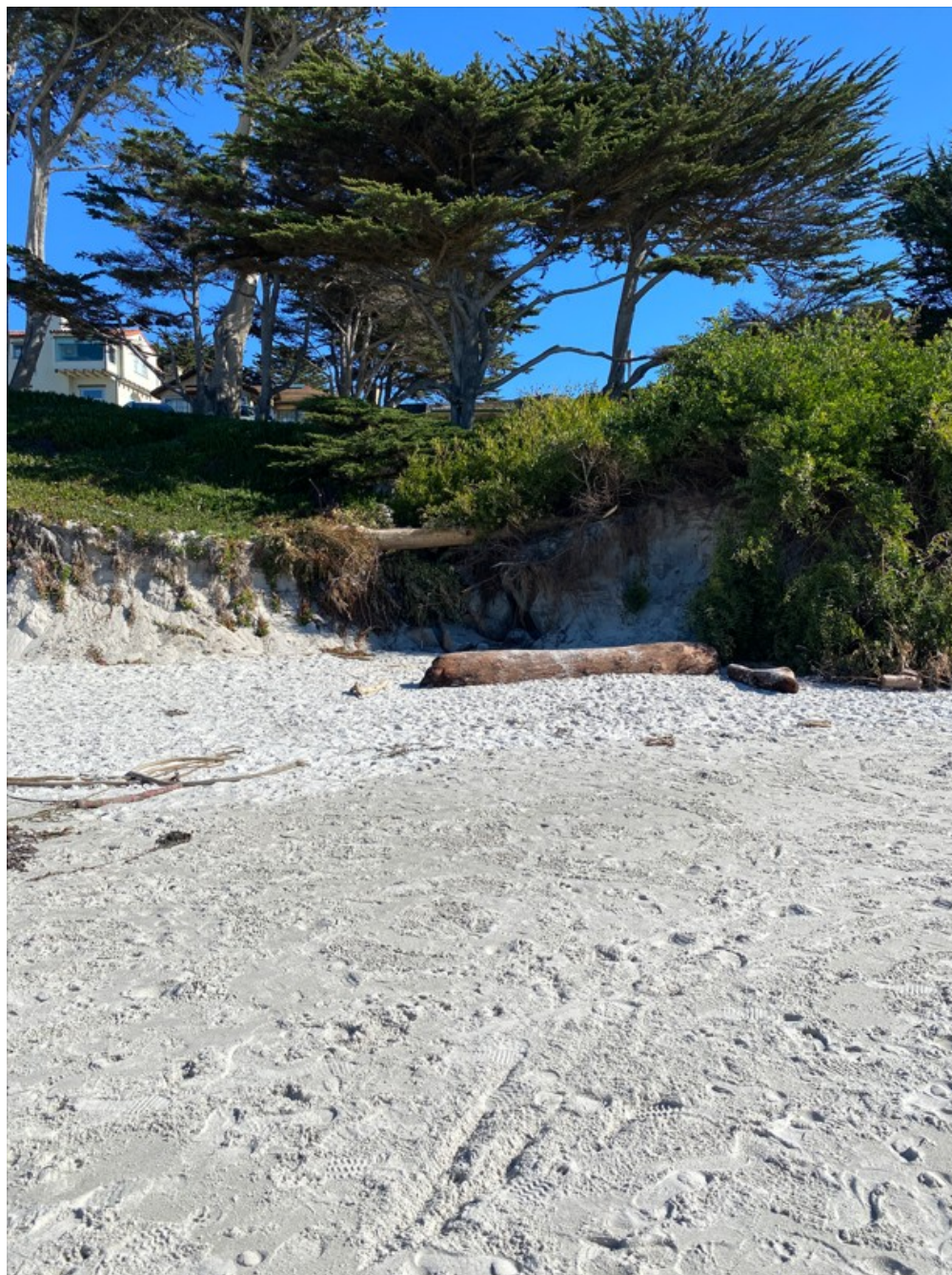
Photograph 81: Small Amount of Revetment R5 Riprap on January 30, 2023
