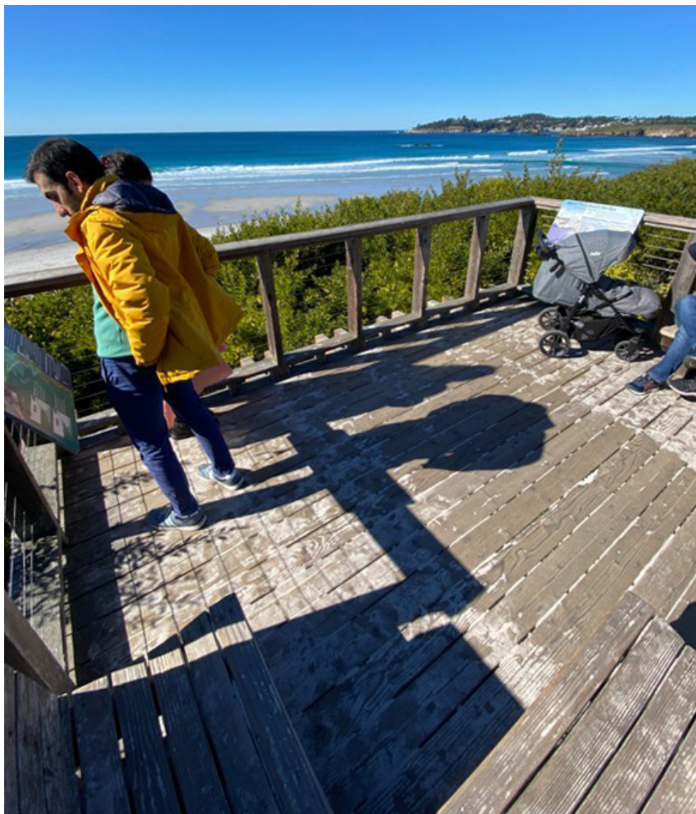
Photograph 90: Stairway ST10 Overlook Platform on January 30, 2023
