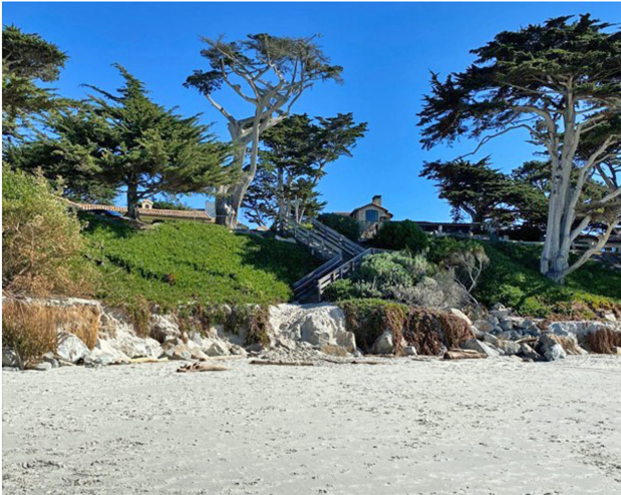
Photograph 79: Showing Beach Access Stairway ST8 on January 30, 2023
