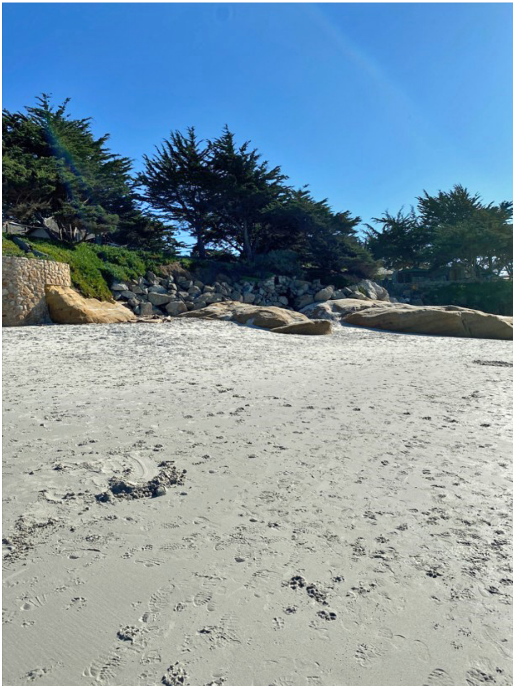
Photograph 20: Showing Revetment R1 and the Southern End of Seawall S3 on January 30, 2023
