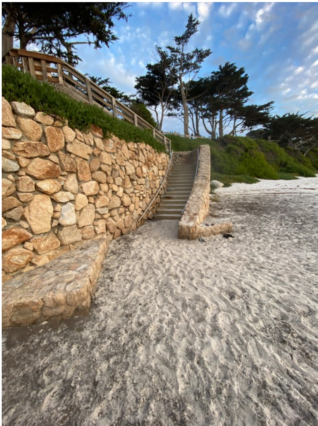
Photograph 64: Showing Stairway ST6 on December 22, 2022
