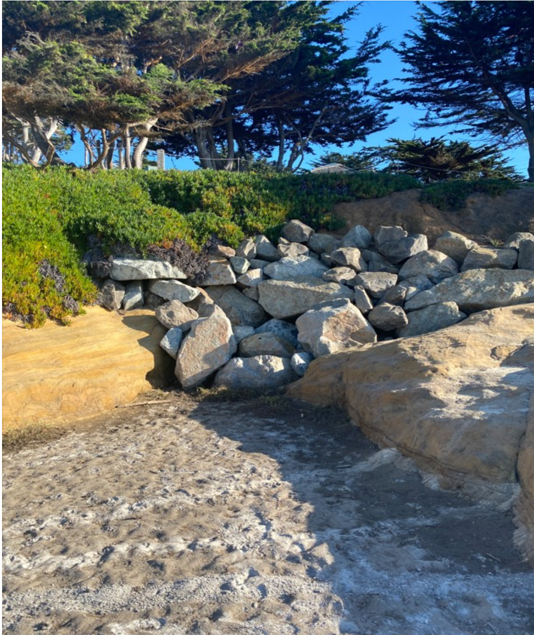
Photograph 19: Revetment R1 on December 22, 2022
