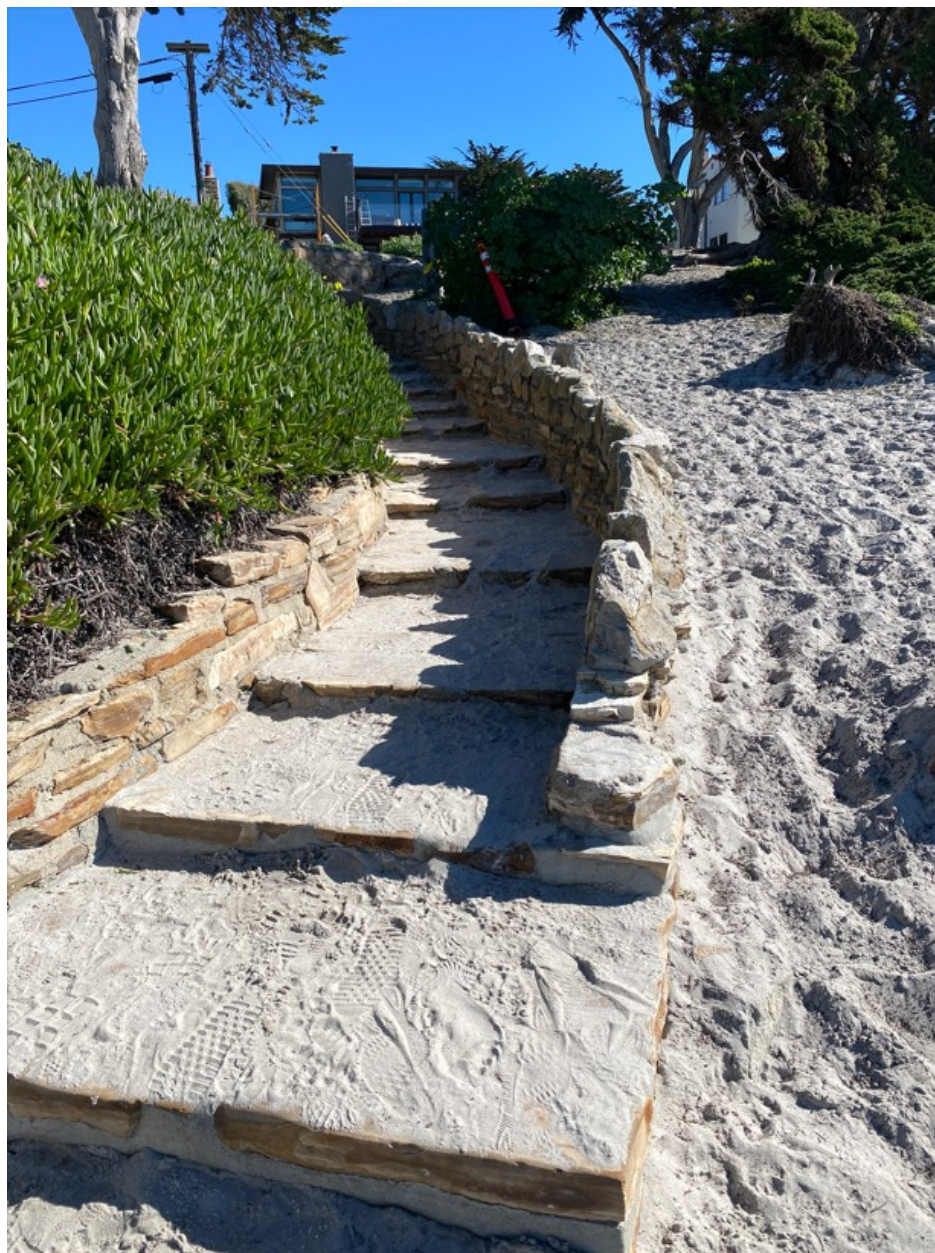
Photograph 86: Stairway ST9 on January 30, 2023
