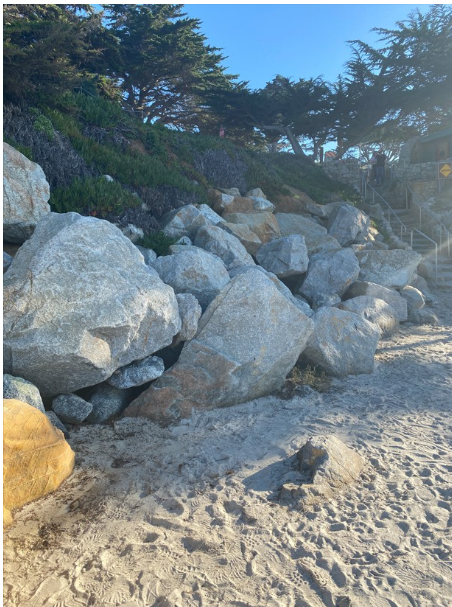
Photograph 17: Revetment R1 on December 22, 2022
