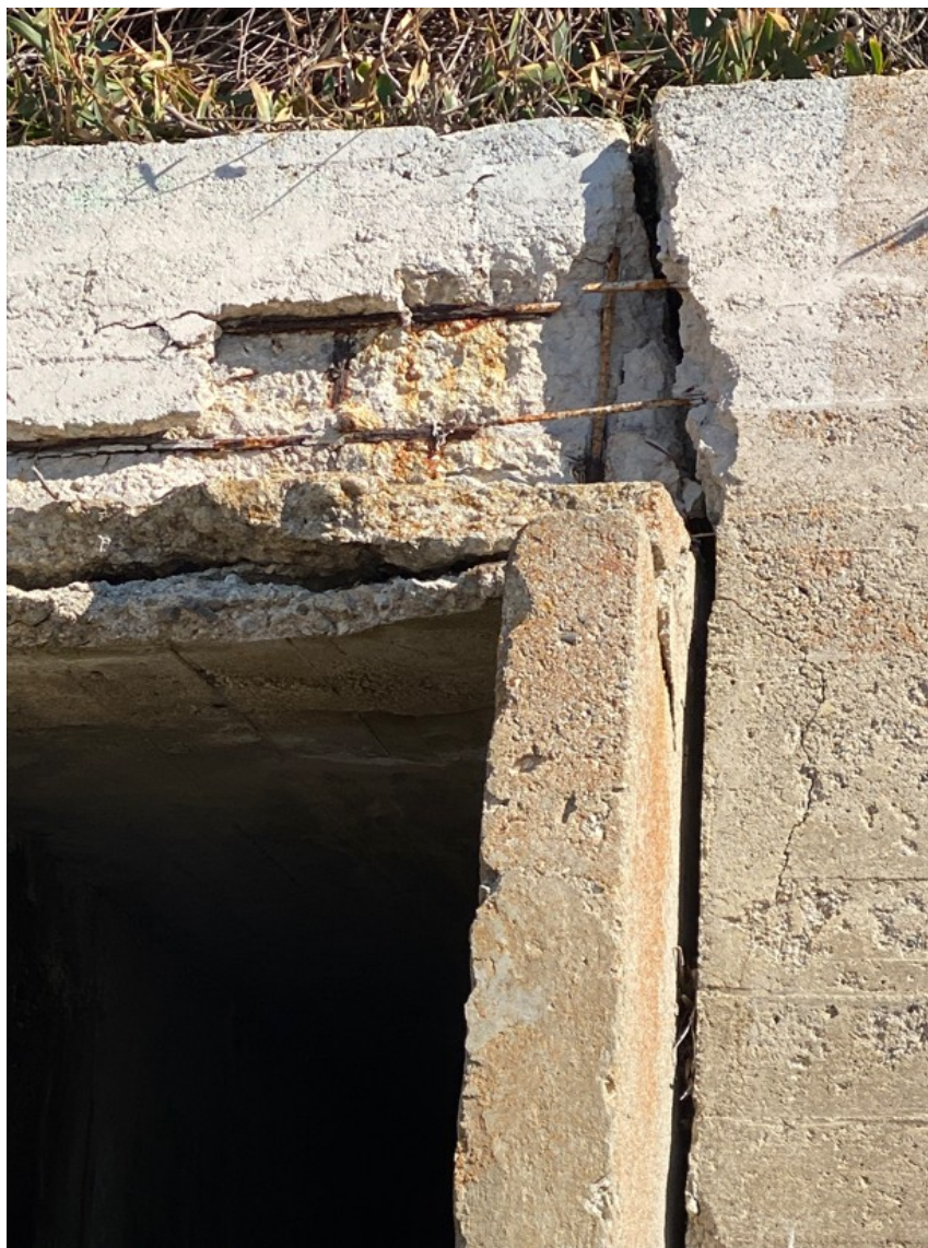
Photograph 95: Seawall S10 on January 30, 2023
