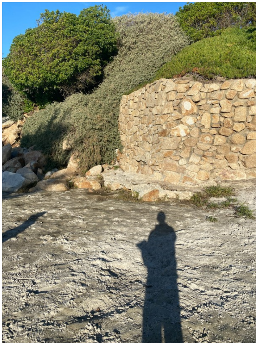
Photograph 32: North End of Seawall S3 on December 22, 2022
