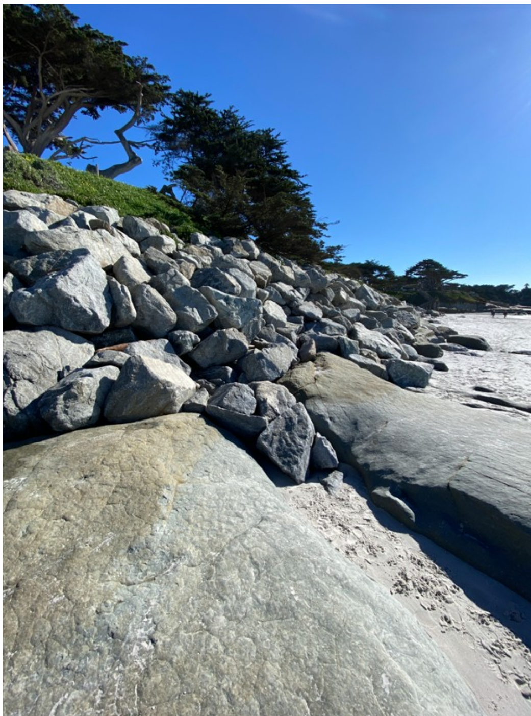
Photograph 53: Profile View of Revetment R3 on January 30, 2023
