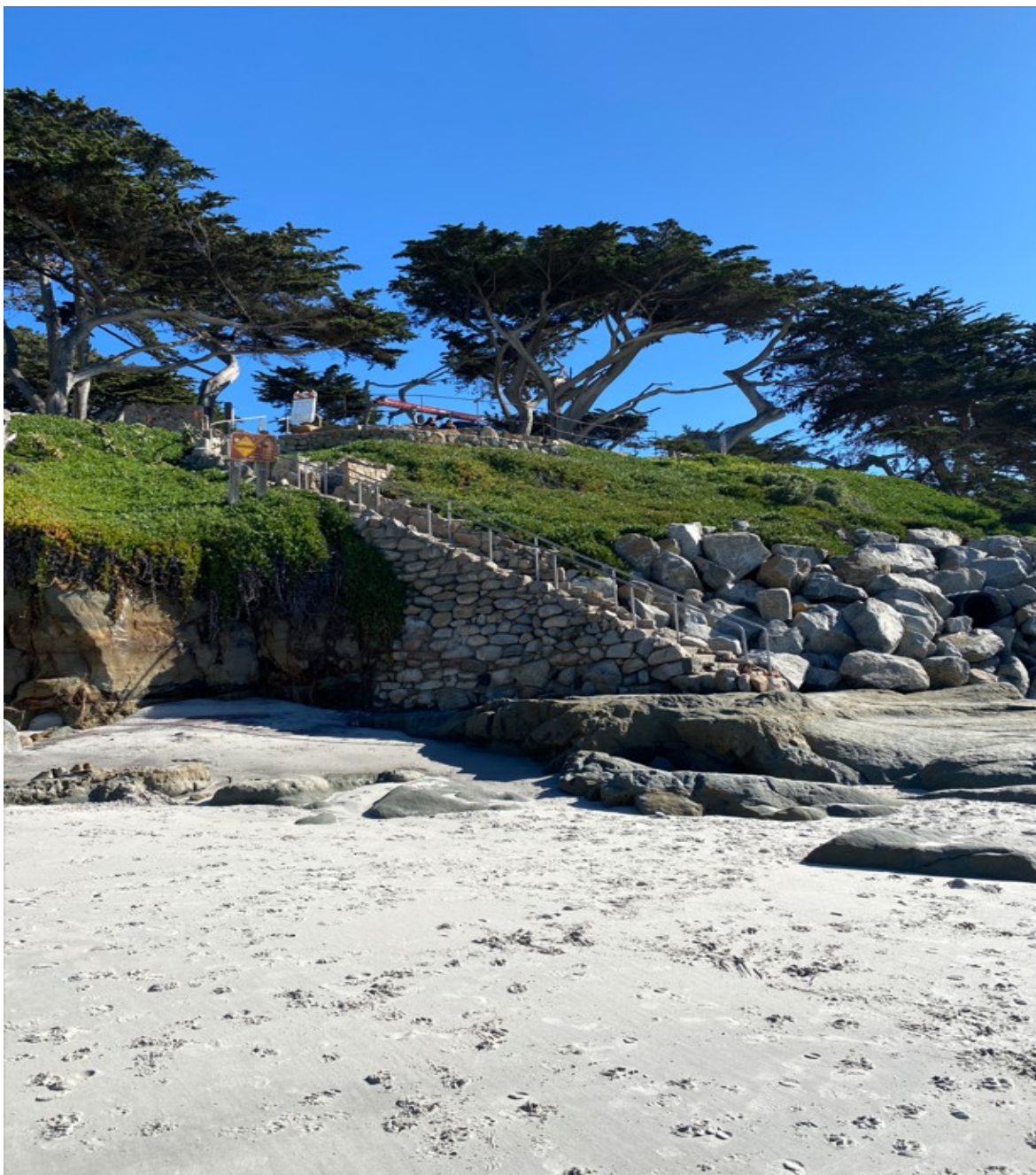
Photograph 56: Showing Stairway ST5 on January 30, 2023
