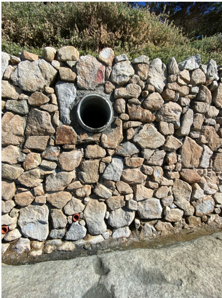
Photograph 69: Storm Drain Outfall near South End of Seawall S7 on January 30, 2023
