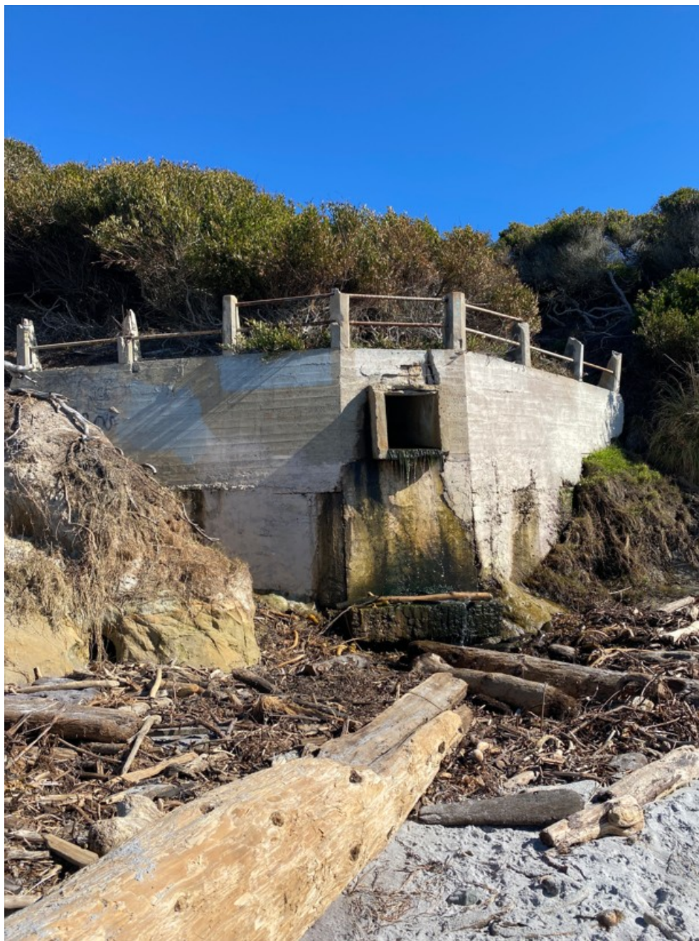
Photograph 92: Seawall S10 on January 30, 2023
