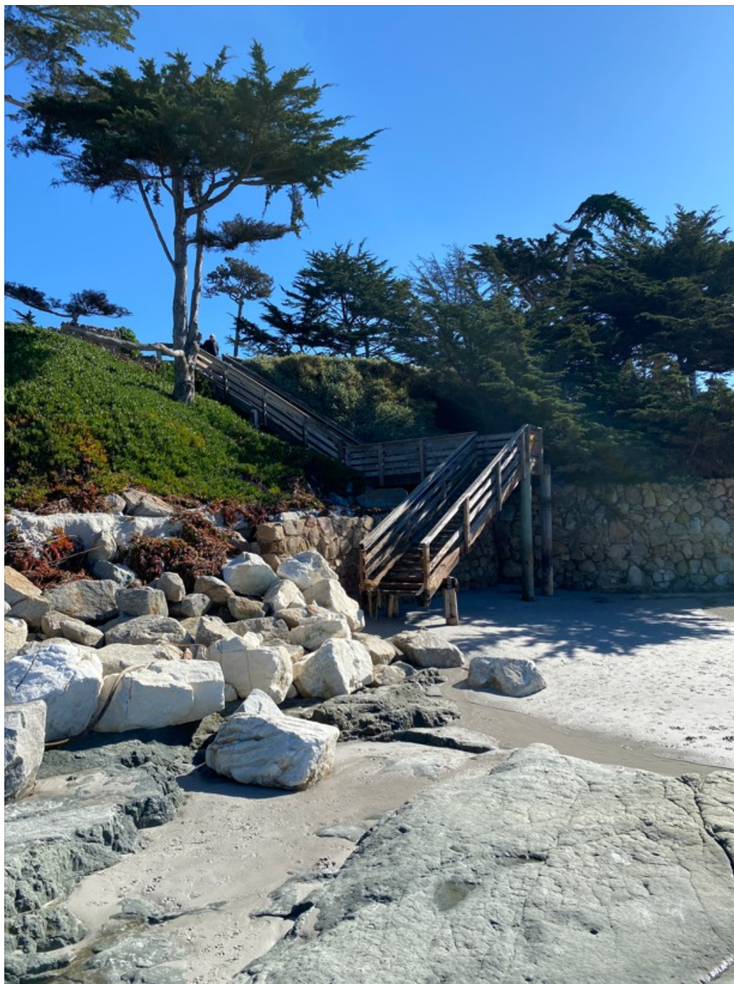
Photograph 73: Stairway ST7 on January 30, 2023
