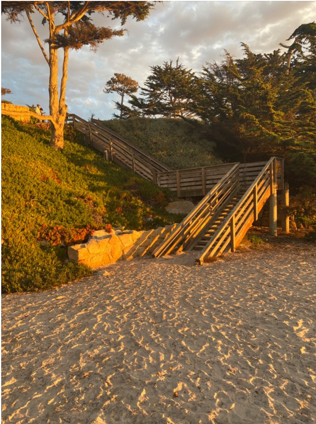
Photograph 72: Stairway ST7 on December 22,2022
